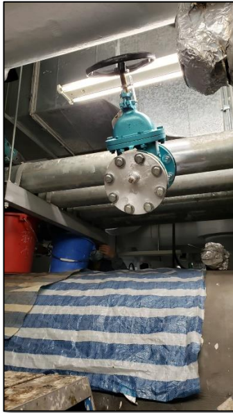
Tie-in Operation Completed
