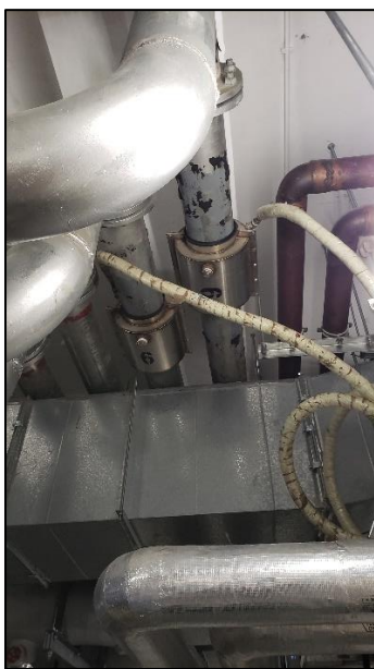
Install pipe freezing clamp
