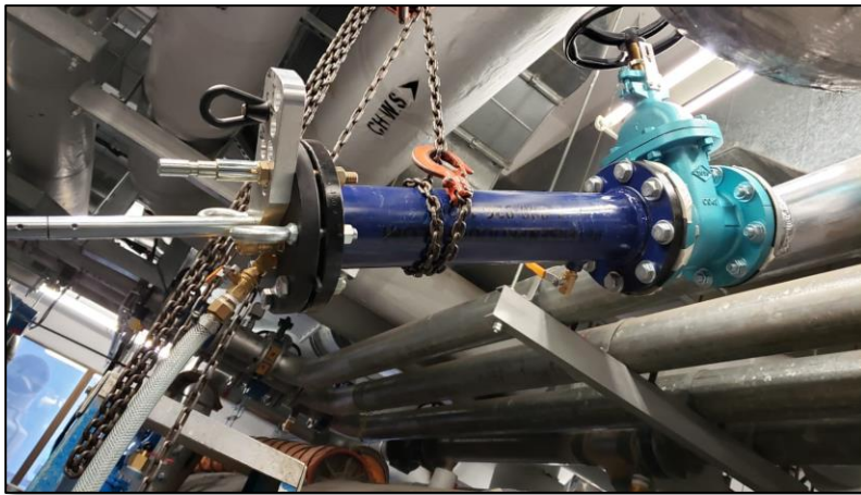
Perform balloon line stop by inflating the balloon
