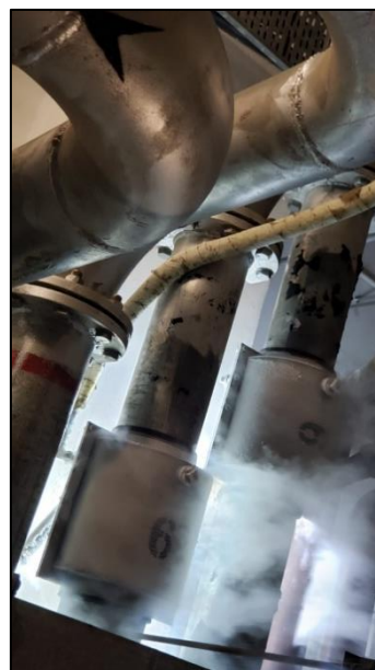
Perform Pipe Freezing
