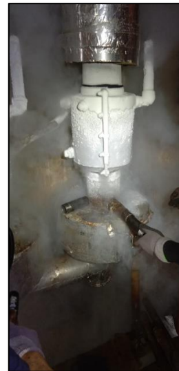
Finish the pipe freezing work
