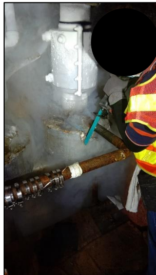
Pipe Freezing at proposed location
