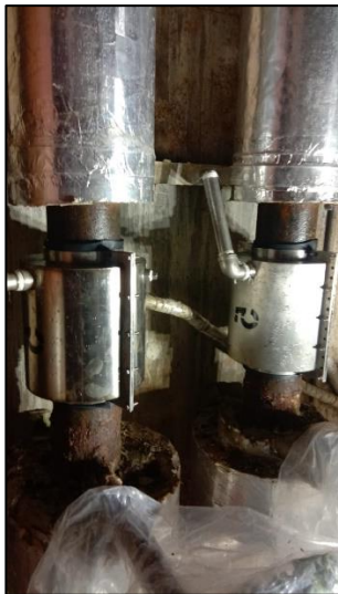
Installation of pipe freezing jacket at proposed location
